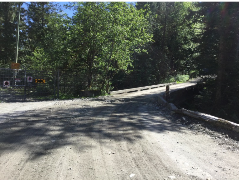
Right Bank Abutment when facing downstream
