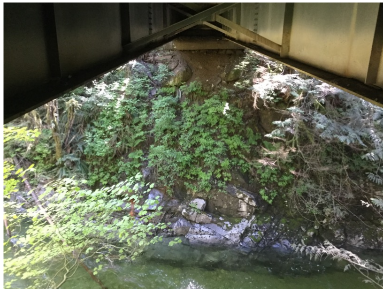
Left Bank Abutment when facing downstream
