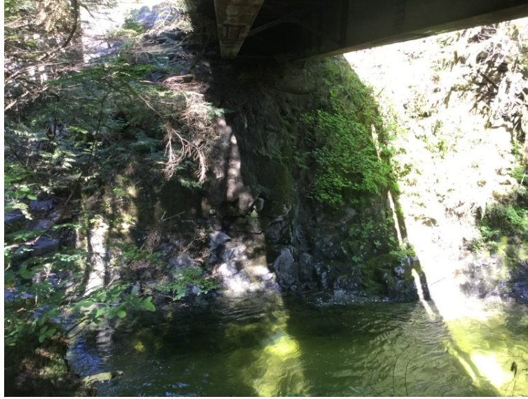
Right Bank Abutment when facing downstream
